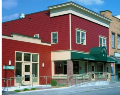
This underutilized pair of commercial buildings in Hamilton, New York, was updated with a whole new color and look, including a new cornice, siding, windows, doors, awning, detailing and other signage. New tenants included offices for a local initiative and a Chinese restaurant relocated from a nearby space. (Source: PlannersWeb)
