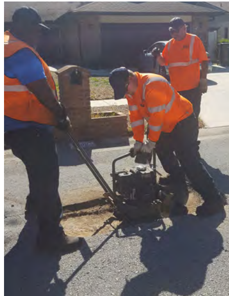
Above: Maintenance crews repair a pothole. L : Maintenance crews replace a drainage culvert pipe.
