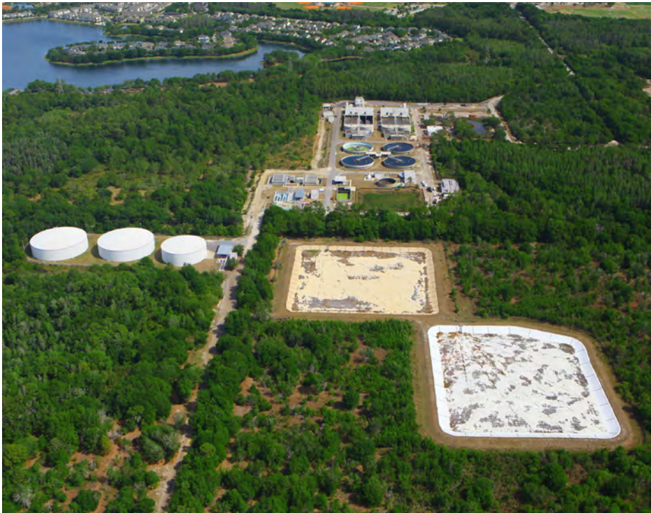
The Northwest Wastewater Treatment Plan will expand to treat wastewater presently treated at the County's Dale Mabry and River Oaks facility.
