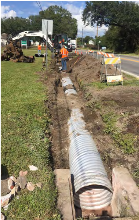
Above: Maintenance crews repair a pothole. L : Maintenance crews replace a drainage culvert pipe.
