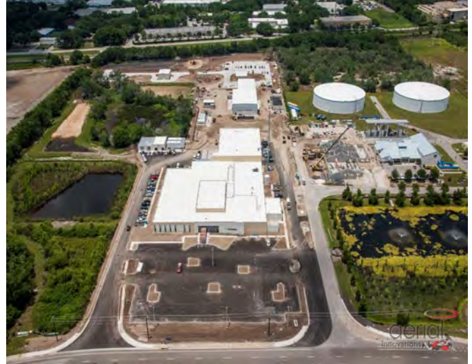
Public Safety Operations Complex (PSOC)
