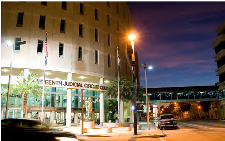
The public entrance to the courthouse complex is through the George Edgecomb Family and Civil Courthouse.
