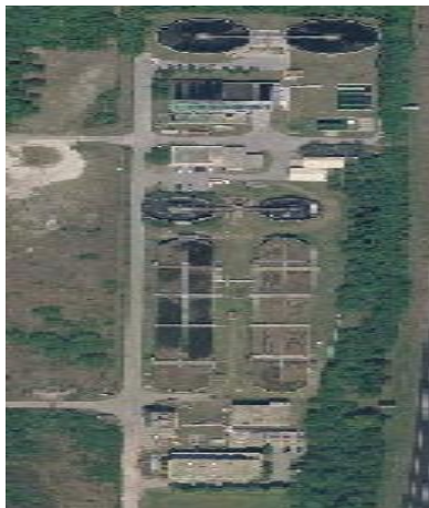
South County AWWTF
