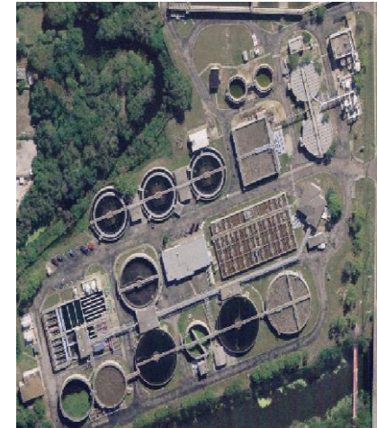
River Oaks AWWTF
