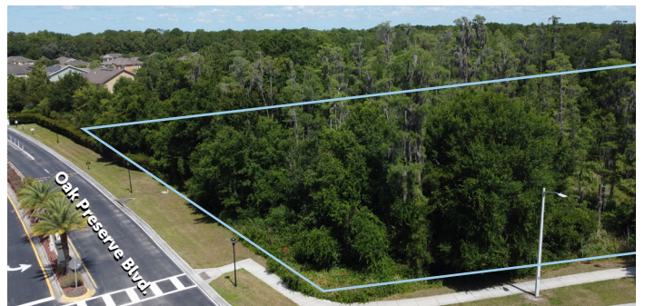
View of Subject Property to the Northwest from Kinnan Street & K-Bar Ranch Intersection
