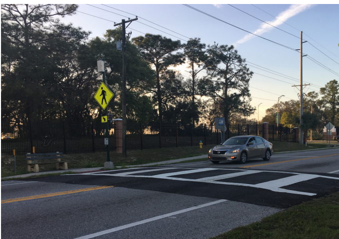
Pedestrian safety enhancements on 50th Street in University area.
