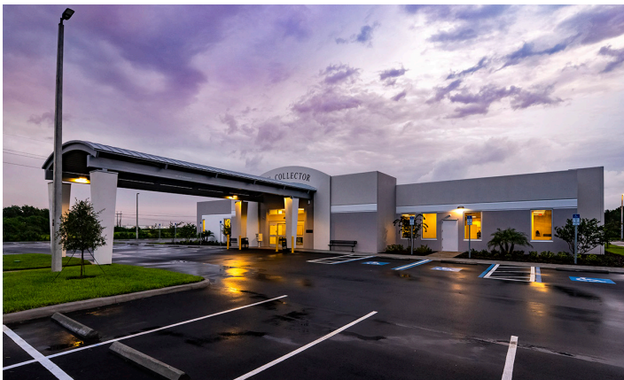
Outside view of our Southshore office – new standard design for Hillsborough County Tax Collector offices.
