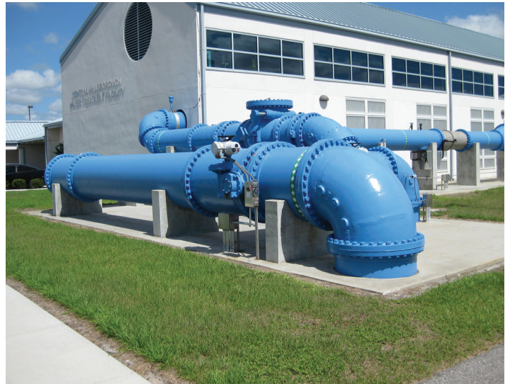
Central Hillsborough Water Treatment Facility.
