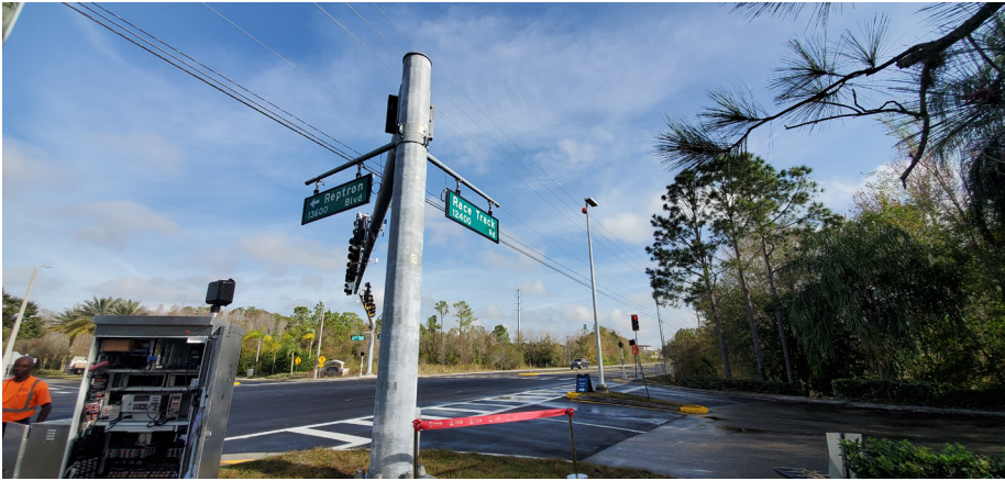
New traffic signal at Repton Boulevard and Racetrack Road.
