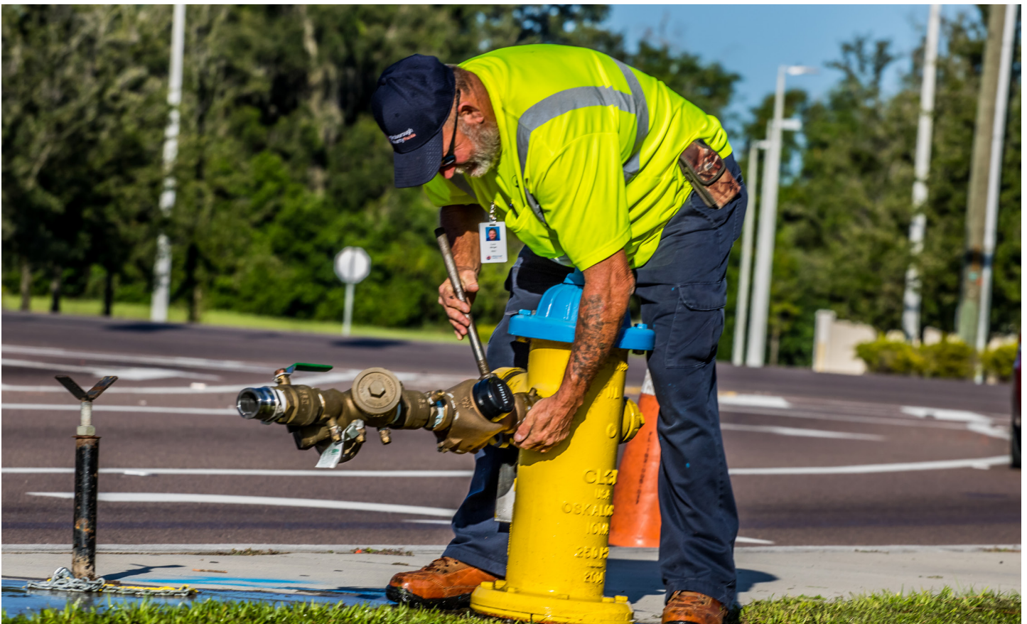
Hydrant Meter Installation.
