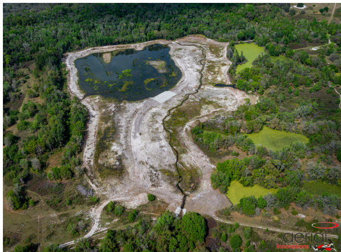
Construction of this 30-acre wetland and stream restoration project at the County's Balm-Boyette Scrub Preserve was completed in December 2019.
