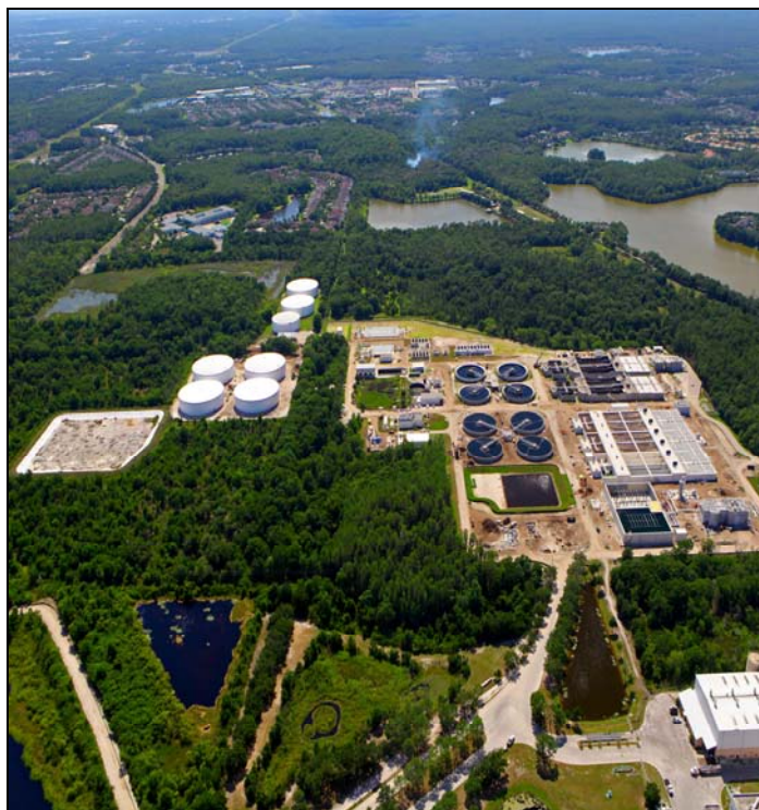
Northwest Regional Water Reclamation Facility System Improvement & Expansion
