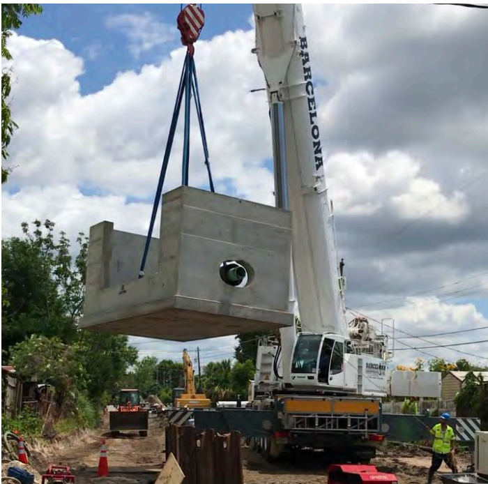
Staff works on Lambright Drainage Project.
