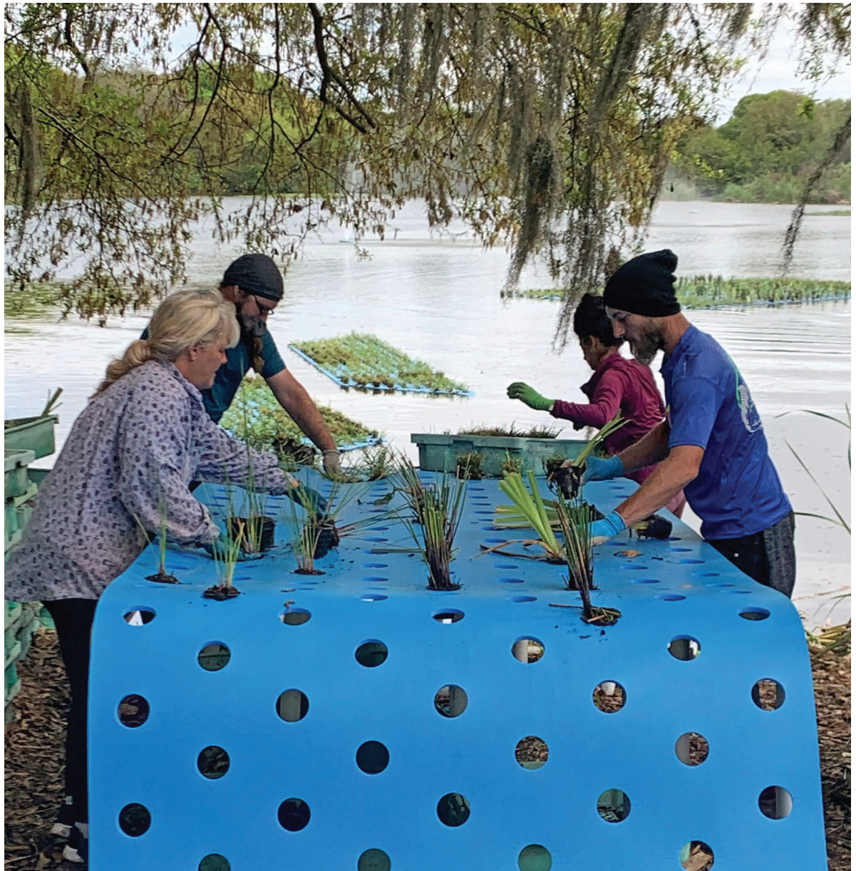
A Floating Wetland Treatment System is installed in a South County stormwater pond.
