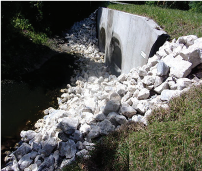
Neighborhood Drainage Improvements
