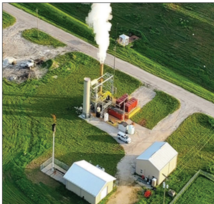
Southeast County Landfill Facility Improvements
