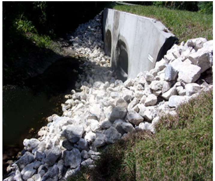
Neighborhood Drainage Improvements
