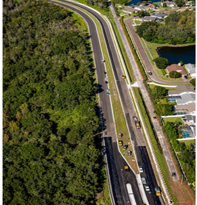
Citrus Park Drive Corridor Improvements
