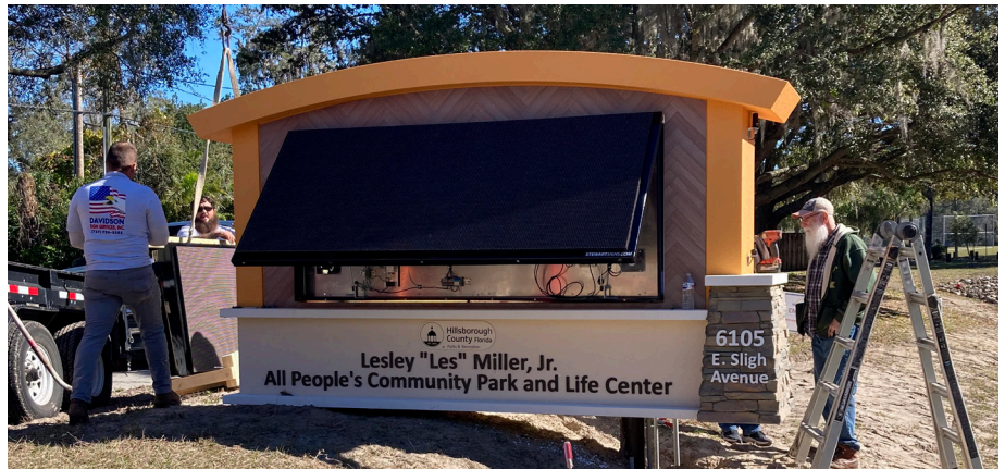
R3M installs the new entrance sign at Lesley "Les" Miller, Jr. All People's Community Park and Life Center.
