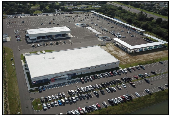
Consolidated and Hardened Maintenance Facility – South Service Unit
