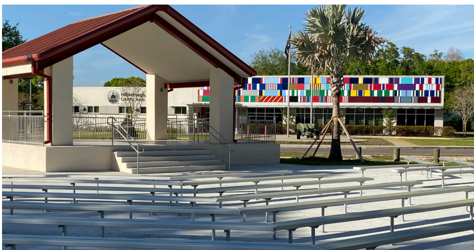
A new amphitheater and gazebo at Veterans Memorial Park provide a wonderful venue for outdoor events.
