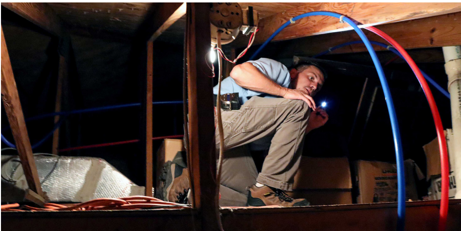
An inspector completes a plumbing inspection.
