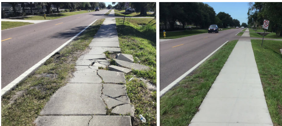
County staff designed and replaced the sidewalk adjacent to the ditch line with reinforcing mat to prevent future erosion issues.
