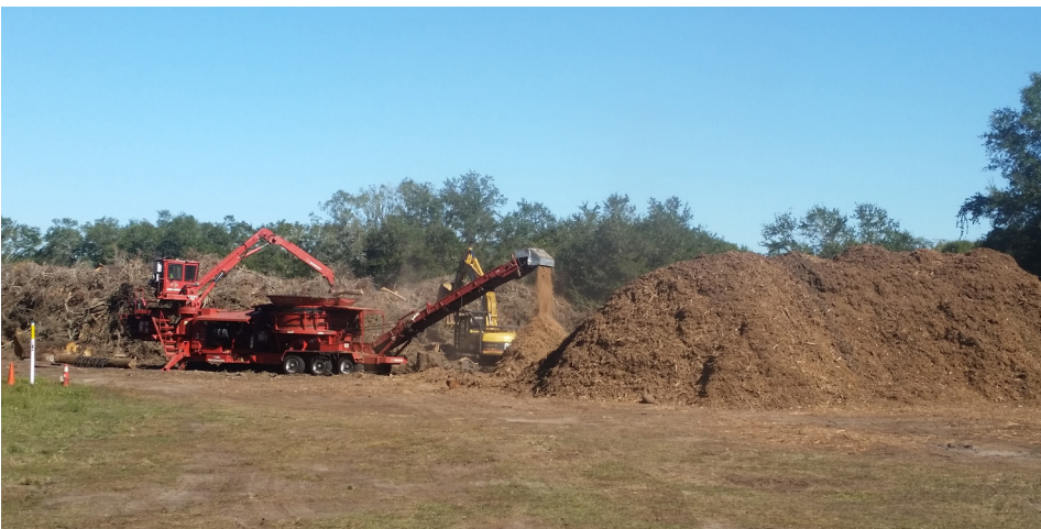
A crew disposes of debris created by Hurricane Irma.
