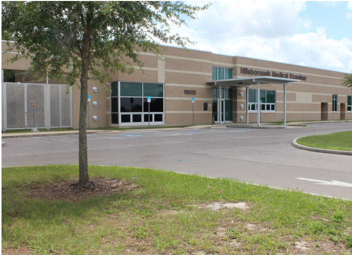
Left: The Medical Examiner Complex Below: Labwork
