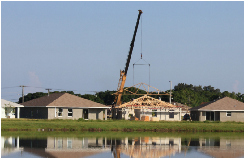
Setting truss on last home in Phase IV
