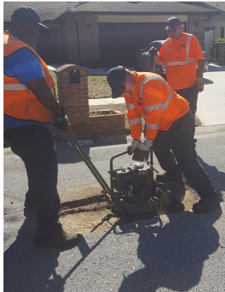
Above: Maintenance crews repair a pothole. Left: Maintenance crews replace a drainage culvert pipe.
