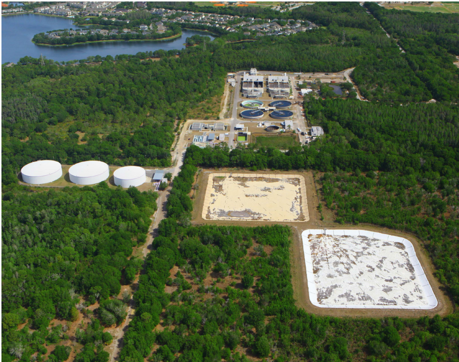
The Northwest Wastewater Treatment Plan will expand to treat wastewater presently treated at the County's Dale Mabry and River Oaks facility.
