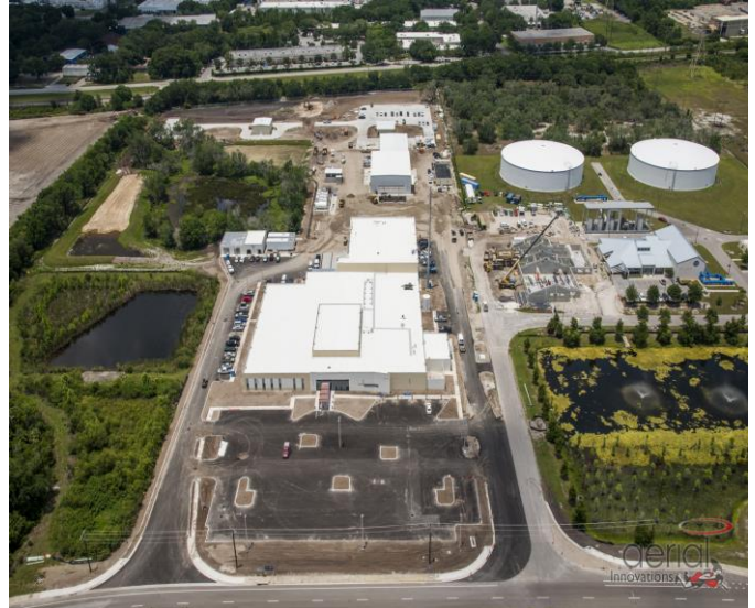
Public Safety Operations Complex (PSOC)
