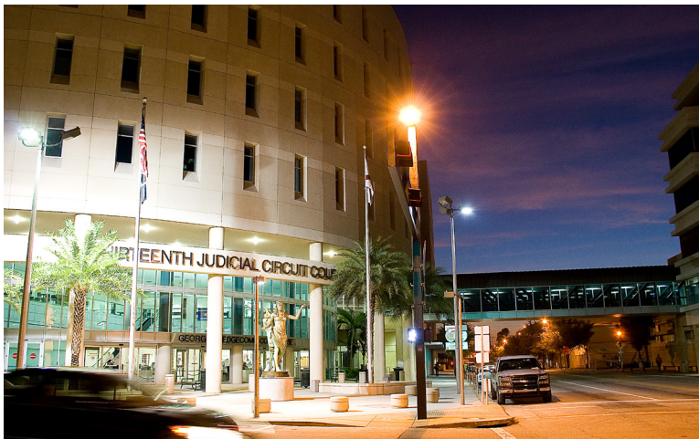
The public entrance to the courthouse complex is through the George Edgecomb Family and Civil Courthouse.
