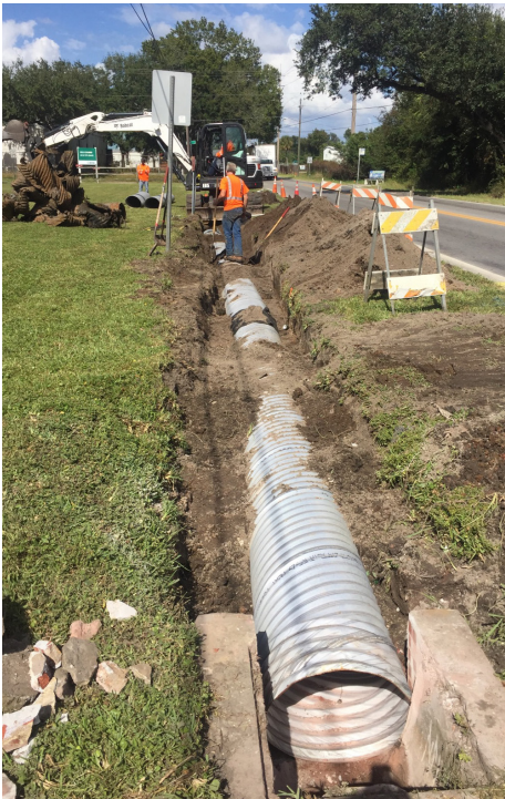
Above: Maintenance crews repair a pothole. Left: Maintenance crews replace a drainage culvert pipe.
