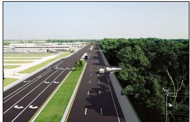
Racetrack Road (After Improvements)
