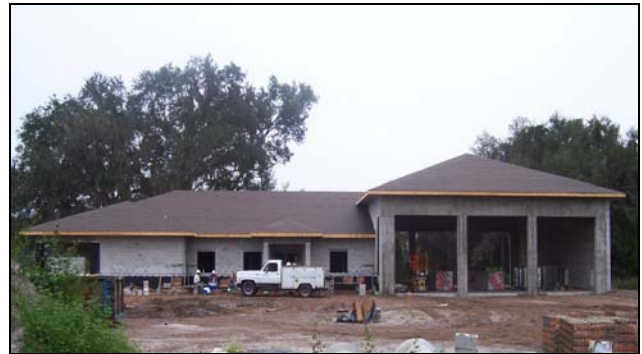
Chapman Fire Station
