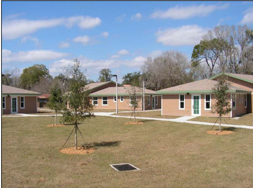
Children Services Campus Enhancements – Dormitories D, E, and F
