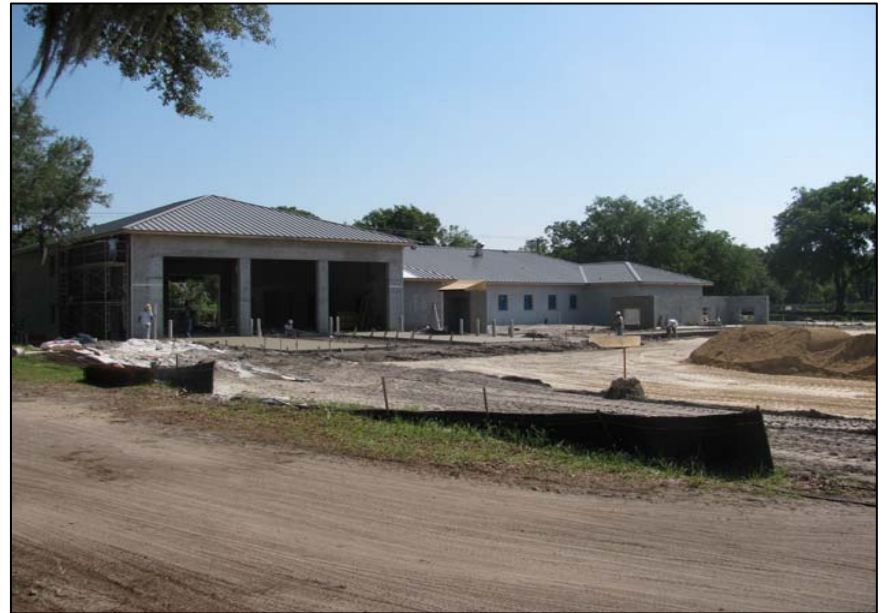
University Area Fire Station #14 (Under Construction)
