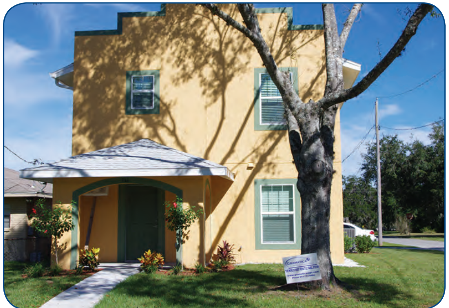
Completion of substantial rehabilitation efforts in University of South Florida neighborhood.
