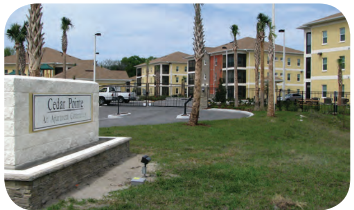
Completion of 60 new multifamily units in the Orient Park NSP Target Area.
