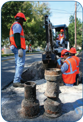
Line Repair Crew
