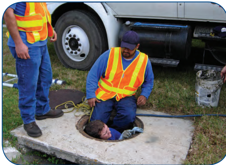
Workers investigate the stormwater pipe system to prepare for maintenance and repairs.
