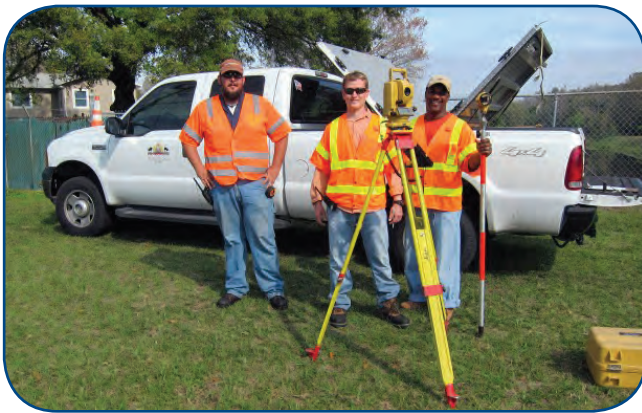
Survey crew in the field preparing for a boundary survey on Falkenburg Road.
