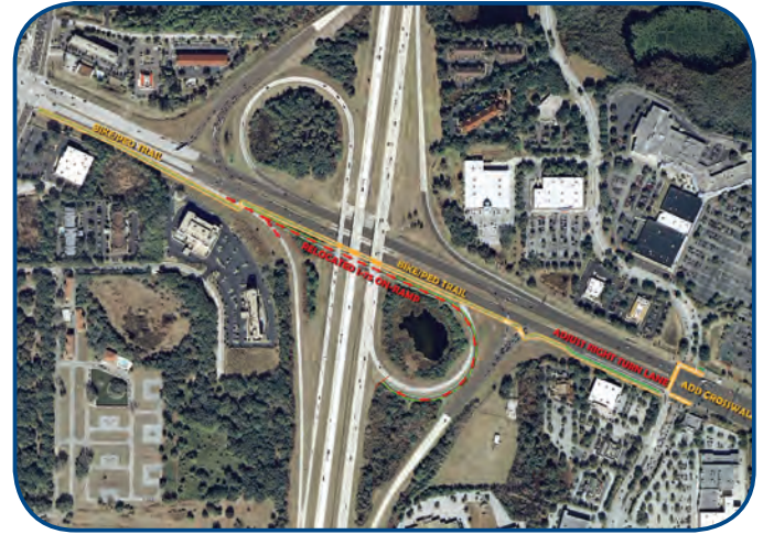
This segment of the Collins Street “Complete Street” is in the historic downtown core.
