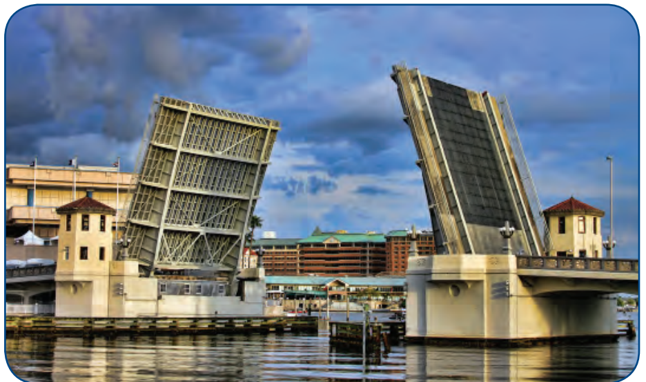
The Platt Street Bridge in downtown Tampa.
