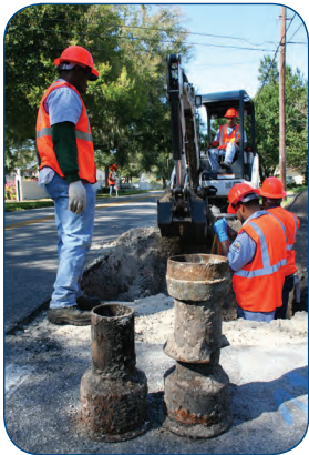
Line Repair Crew
