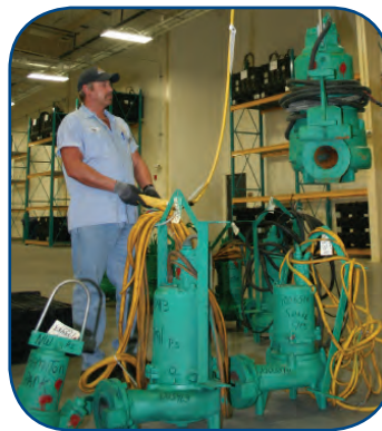
A staff member puts in a hard day's work in the submersible pump maintenance shop.
