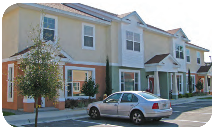
New housing construction of a town home community called Alexander Wood.
