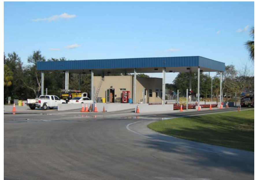
Resource Recovery Facility Scale House Replacement and Entrance Road Improvements Project
