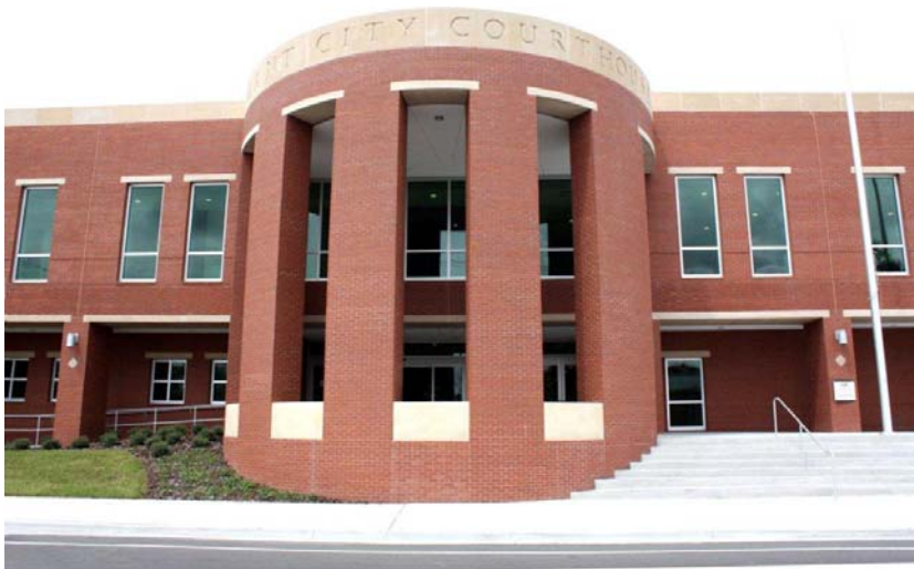
East County Court Redevelopment Project
