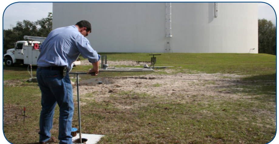
A staff member conducts valve maintenance for the County's drinking water system.
