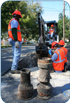
Line Repair Crew
