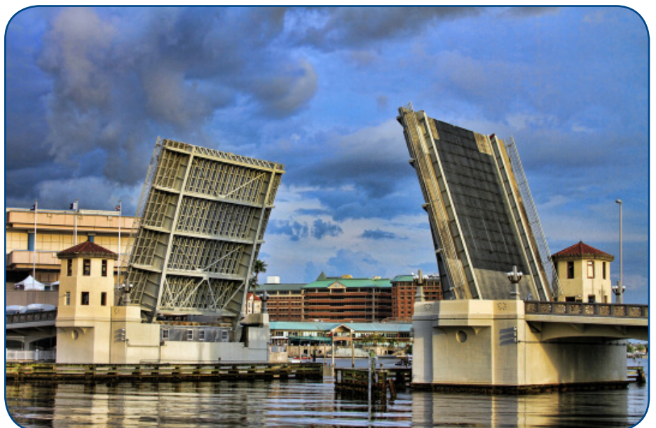
The Platt Street Bridge in downtown Tampa.
