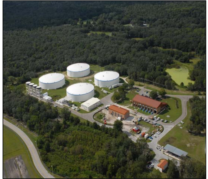
Lithia Water Treatment Plant
