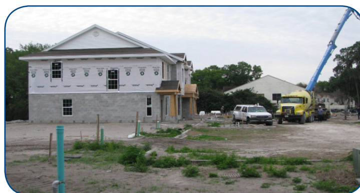
Construction takes place for Alexander Woods new eight-unit townhomes.
