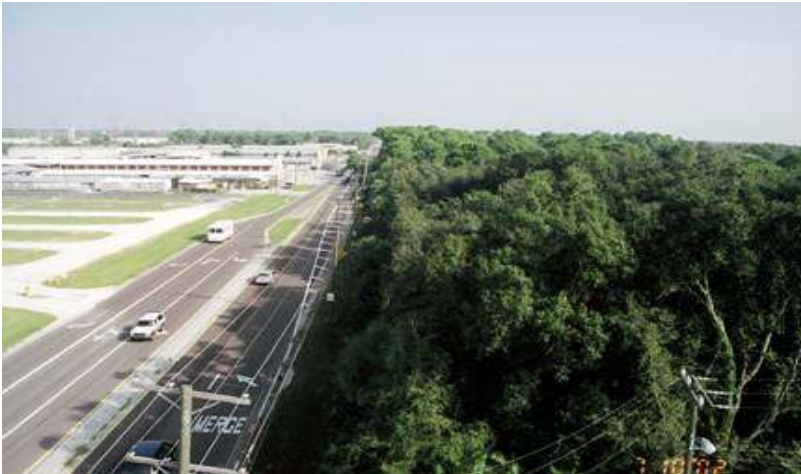
Racetrack Road (Before Improvements)
