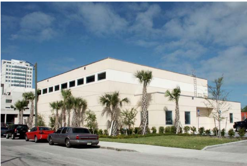
New Chiller Plant
