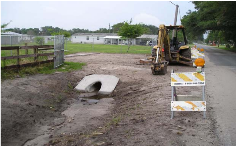
Clay Turner Road Stormwater Improvements
