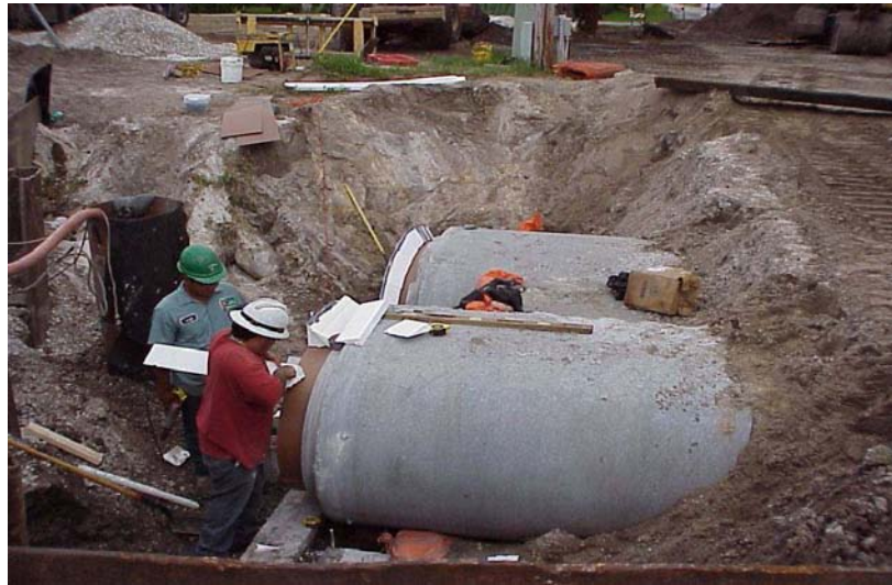
County workers install new reinforced concrete pipe to improve stormwater drainage
