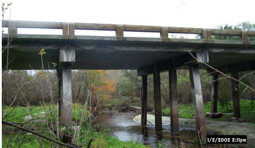
Lithia Pinecrest Bridge
