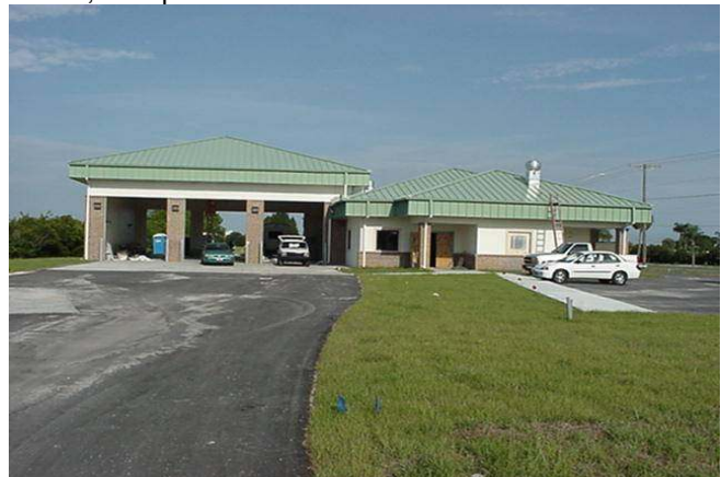
New Sun City Fire Station (Under Construction)
