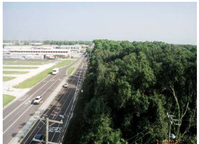
Racetrack Road Before Improvements
