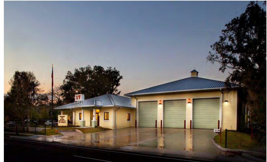
Ruskin Fire Station #17
