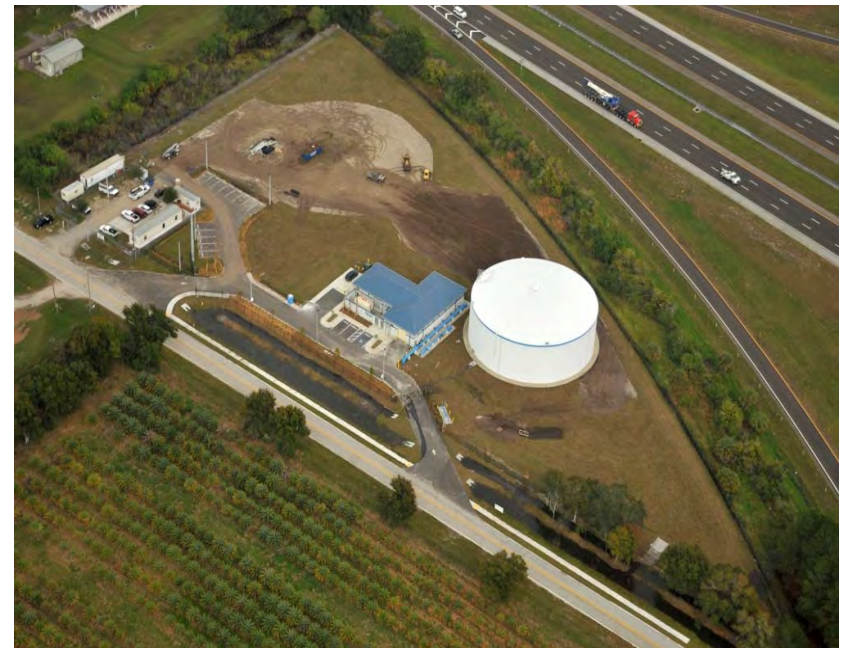
South County Potable Water Repump Station Project
