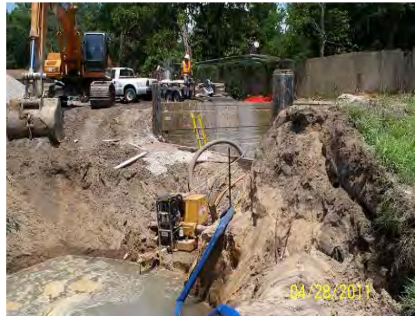
East Morgan Retention Pond
