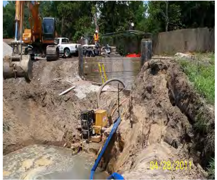
East Morgan Retention Pond
