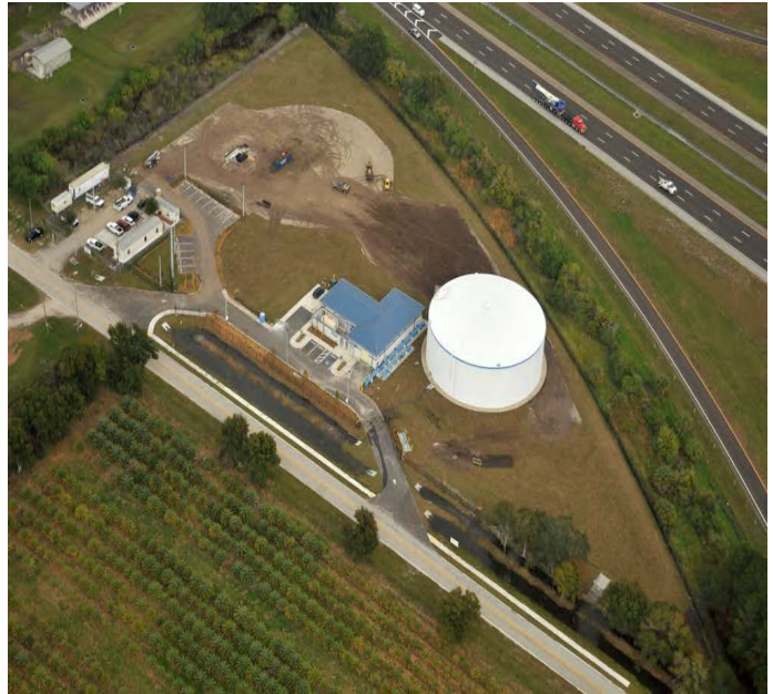
South County Potable Water Repump Station Project
