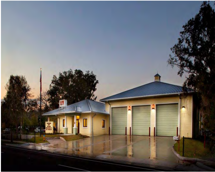
Ruskin Fire Station #17
