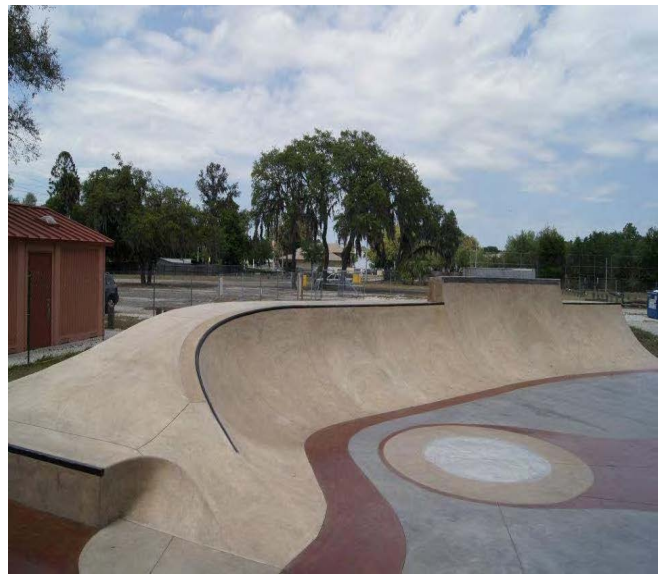
Brandon Skateboard Park (Completed in February 2012)
