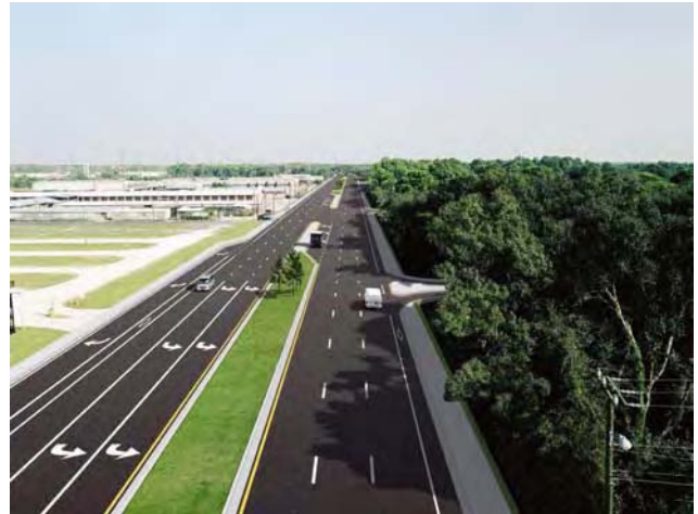
Racetrack Road (After Improvements)
