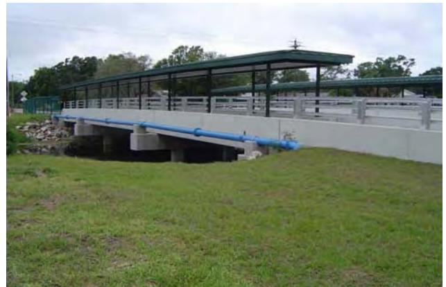
Completed Webb Road Bridge Replacement
