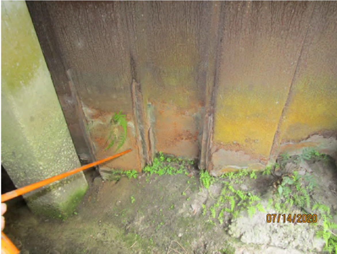
Photo 1: Element 8474 Metal Wall
